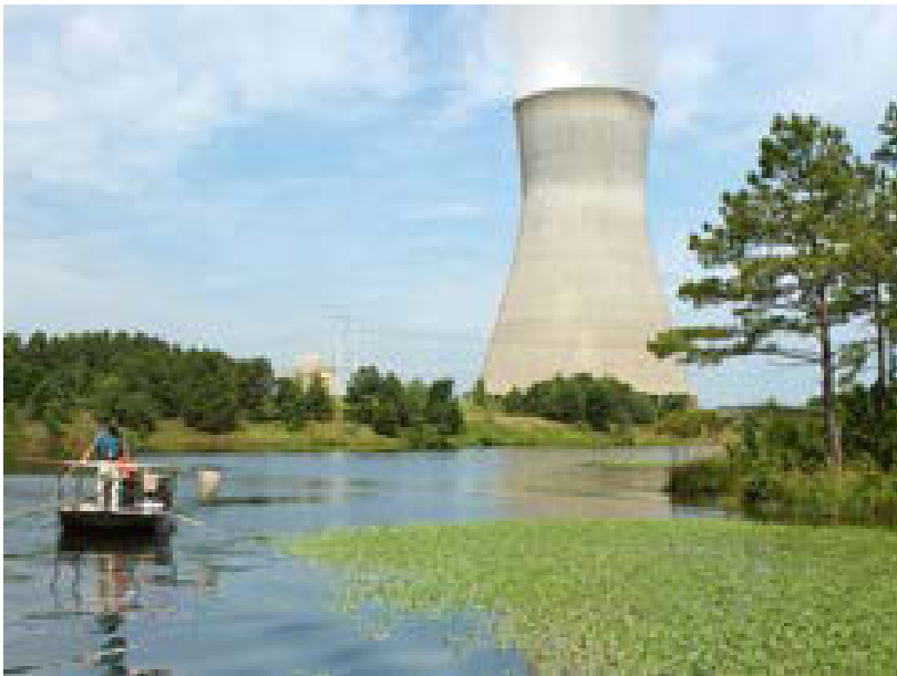
Figure 3-53: Harris Nuclear Plant
