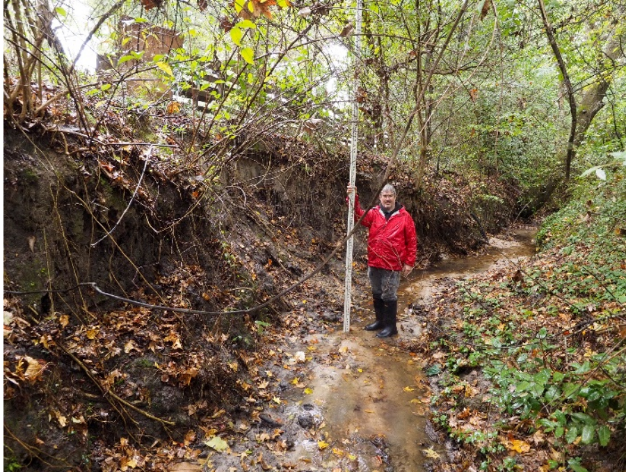
Figure 7. Threatened private fence and outbuilding (visible at top left)
