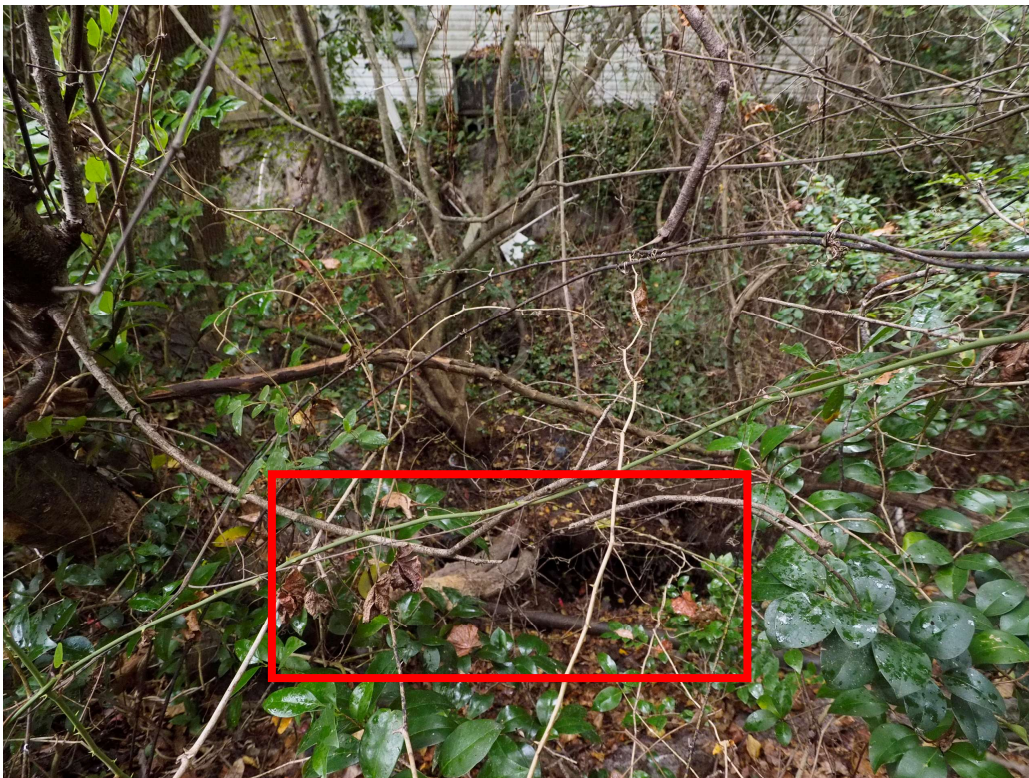
Figure 5. Exposed Steel-Cased Electric Service Line
