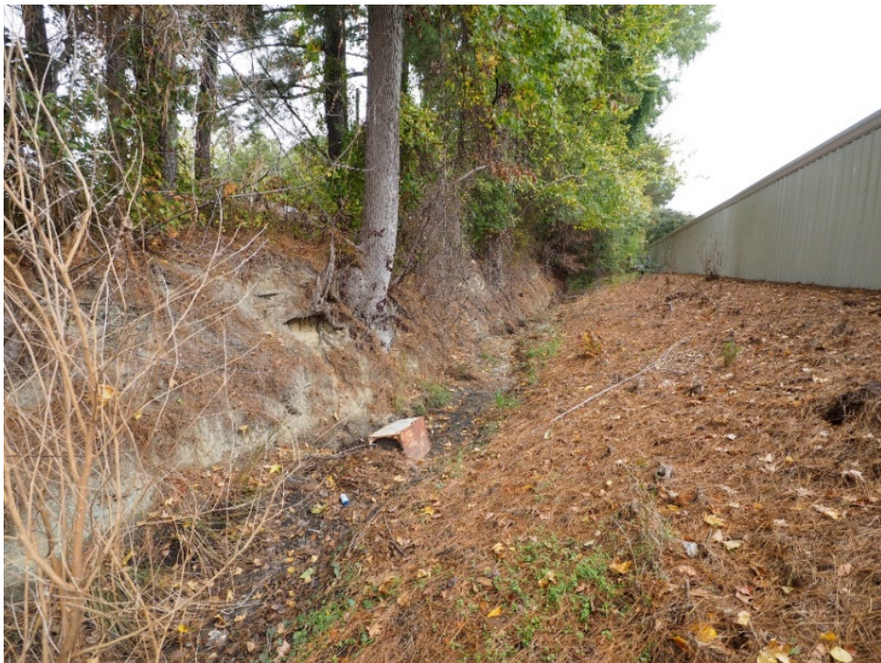
Figure 2. Graded floodplain bench and 2:1 tie-in grading.
