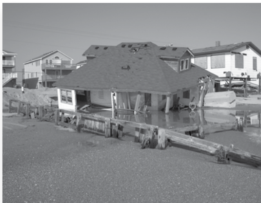
Dare County home destroyed by Hurricane Isabel
