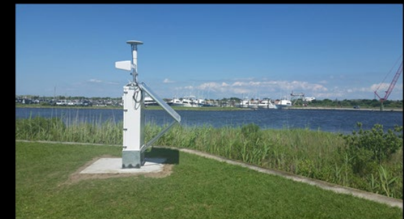
Solar Powered CORS at Oregon Inlet
