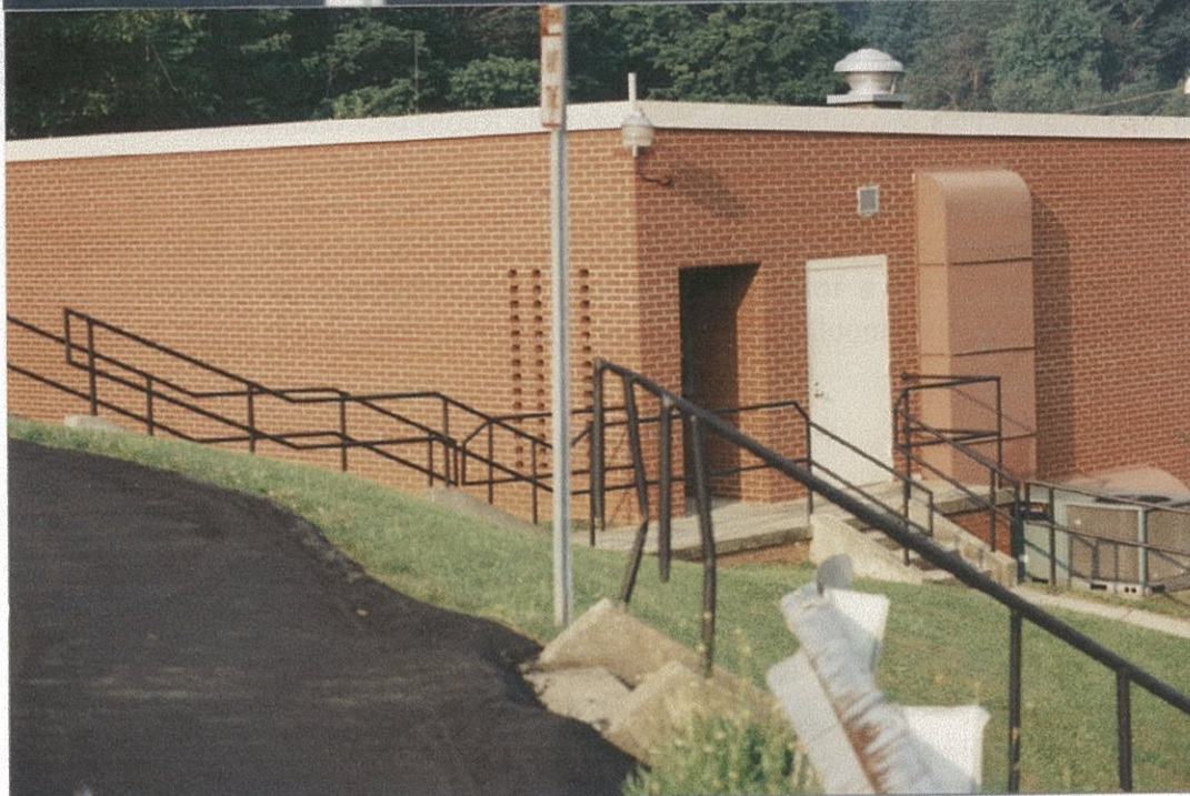
Top: Entrance to the second home of Asheville Radio, located to the rear of Troop "G" Headquarters building. Troop "G" ComCenter operated from this building from October 1953 to October 1980. Photo taken 14 June 1995.
