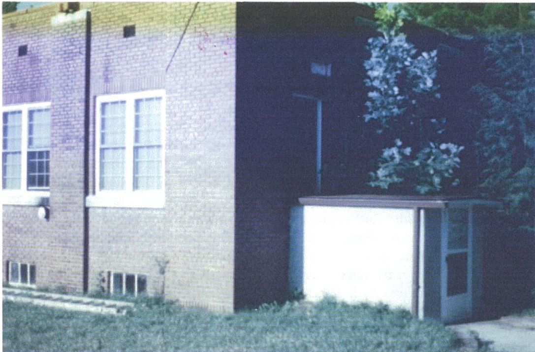
The East and rear view of old Radio Station WANJ, Swannanoa, N. C., across the street from Owen Middle School. Photo taken 6-14-95
