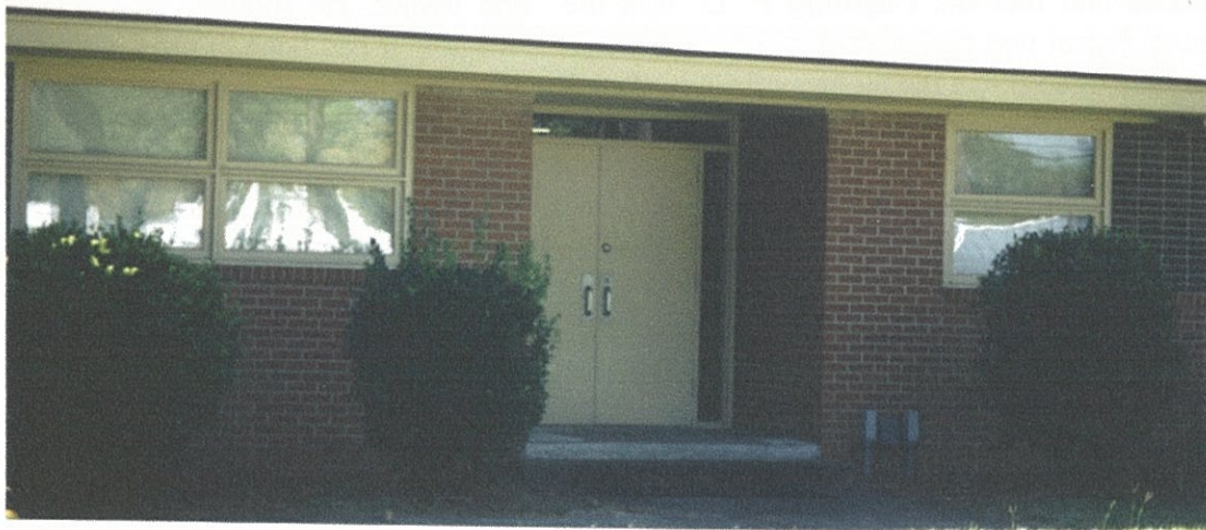
Top Photo: New Hanover County Courthouse, Princess Street Annex, Wilmington, NC. SHP Radio Station KIB-365 was located next to the first floor window on right from 1949 to 1959.
