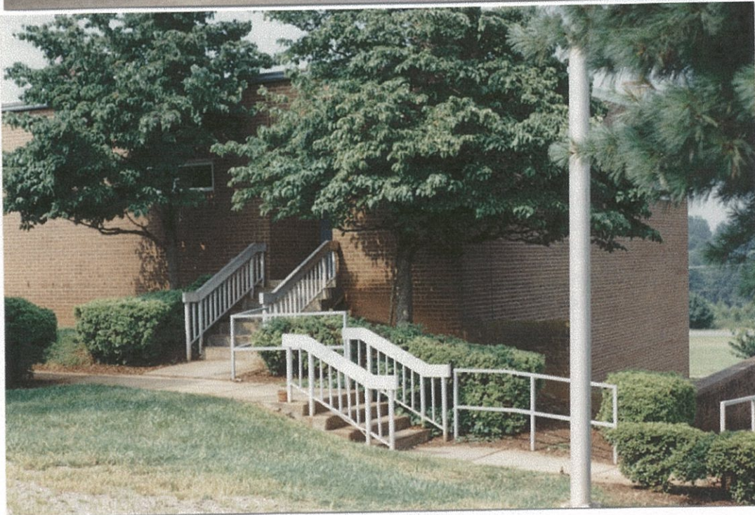
Top: Looking SE at Troop "F" Communications Center First floor occupied by Radio Maintenance & Repair Shop Photo taken 16 May 1998 Bottom: Entrance to second floor of Troop "F" ComCenter Photo taken 17 July 1995
