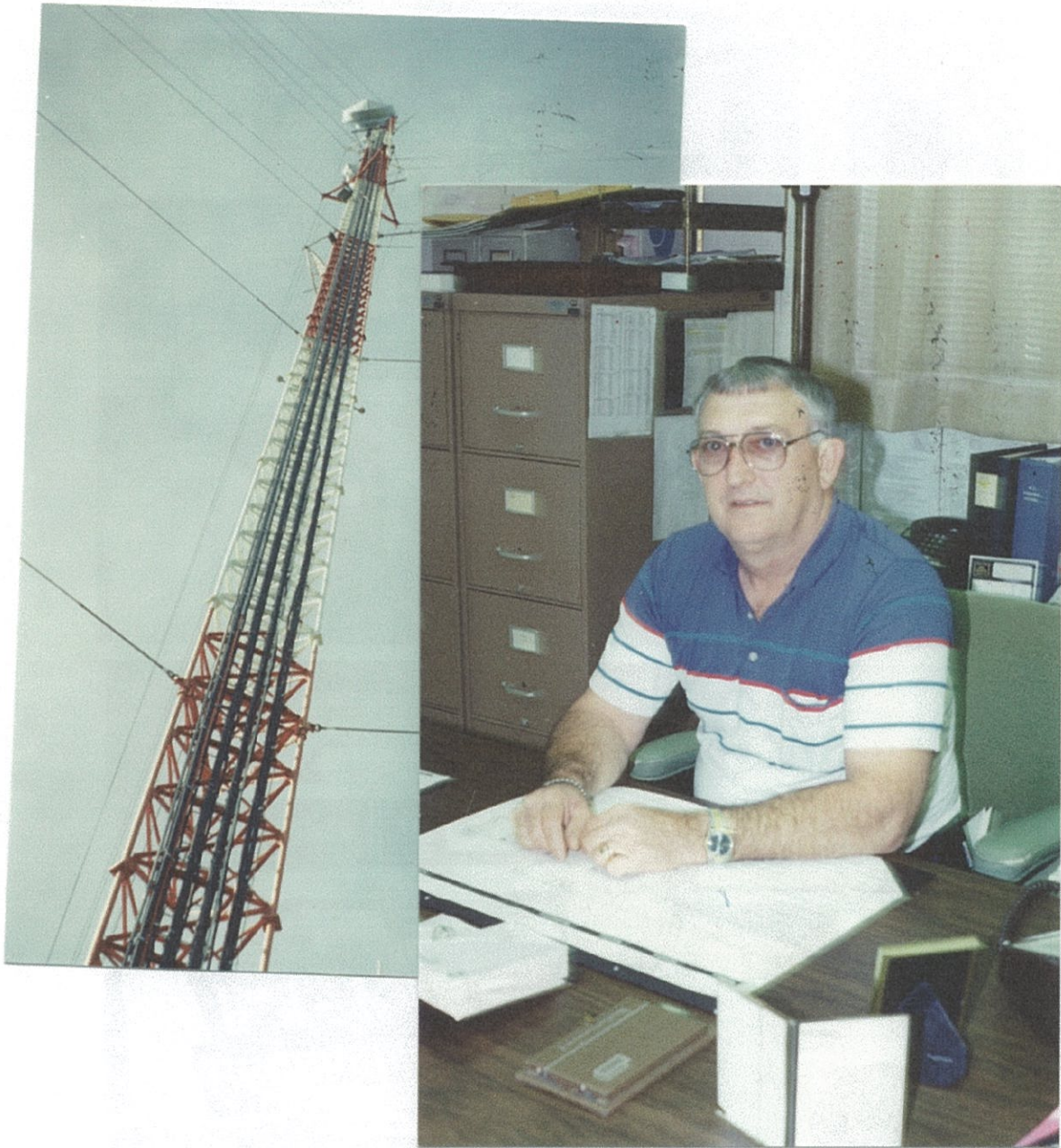
Left: Troop "A" ComCenter base antenna tower, located within a few hundred feet South of the station building.
