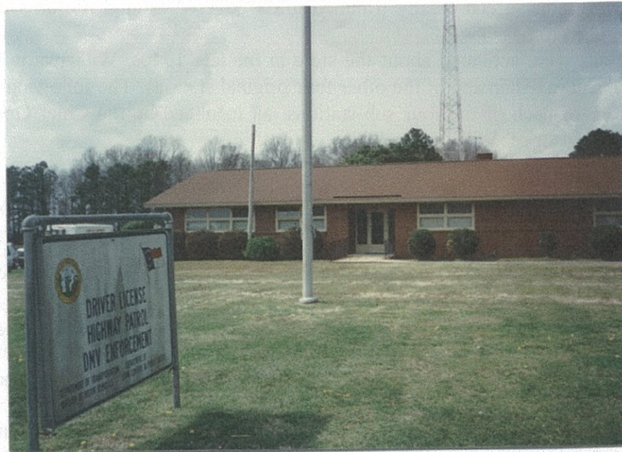
This was the third home of Elizabeth City Radio WFGX/KIA-615 1963-1974. It continues to be used by the State Highway Patrol as a District office, Driver License Examiners, and DMV Inspector office. Photo by Harold Riddick, former Telecommunicator at Elizabeth City, who retired in 1995 as the Center Supervisor of Troop "A" Communications Center, Williamston, North Carolina.
