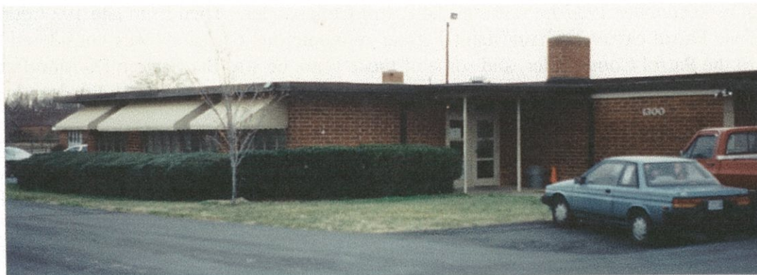
Headquarters- C & L Complex 1300 Blue Ridge Road Raleigh, NC
