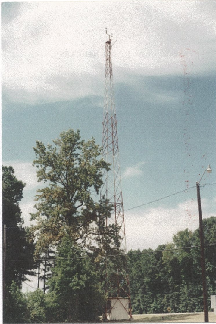
Base tower for Radio Station KIB-900, (formerly WLTI) Rocky Mount, NC The station building stood a few feet to the right of the tower. This tower is now utilized by Troop "A" Communications Center as a repeater station. Photo taken 20 August 1995
