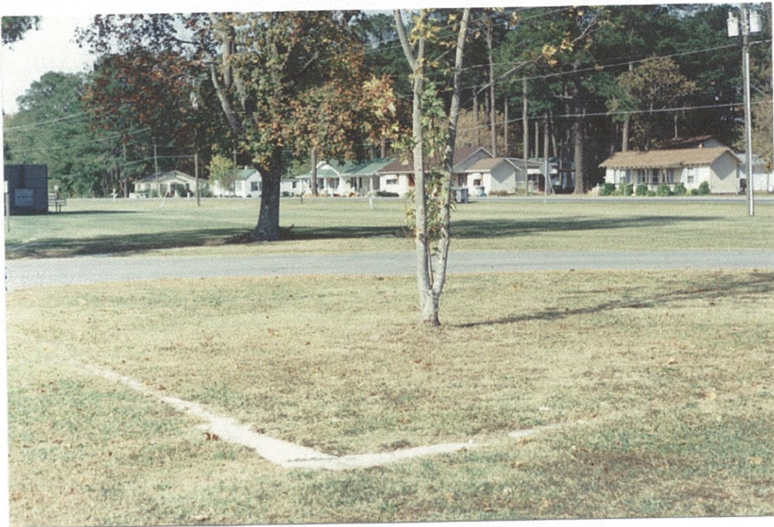
Site of Radio Station WANI. Portions of South and East foundations are shown with a tree planted inside the area where the building once stood. Photo taken 2 November 1994
