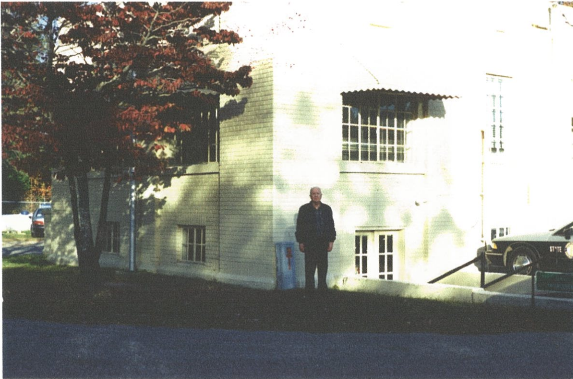
Retired Radio Engineer II John W. Baird, standing at the SW corner of the original building of Radio Station WANL, one of three of the original five such buildings still standing today. This historical structure, built in 1936-1937, was well maintained when the author visited and made this photo on 7 November 1994. The building and surrounding premises are still owned by the State of North Carolina, and is presently occupied by the Enforcement Division of the State Highway Patrol, and Driver License Examiners offices.
