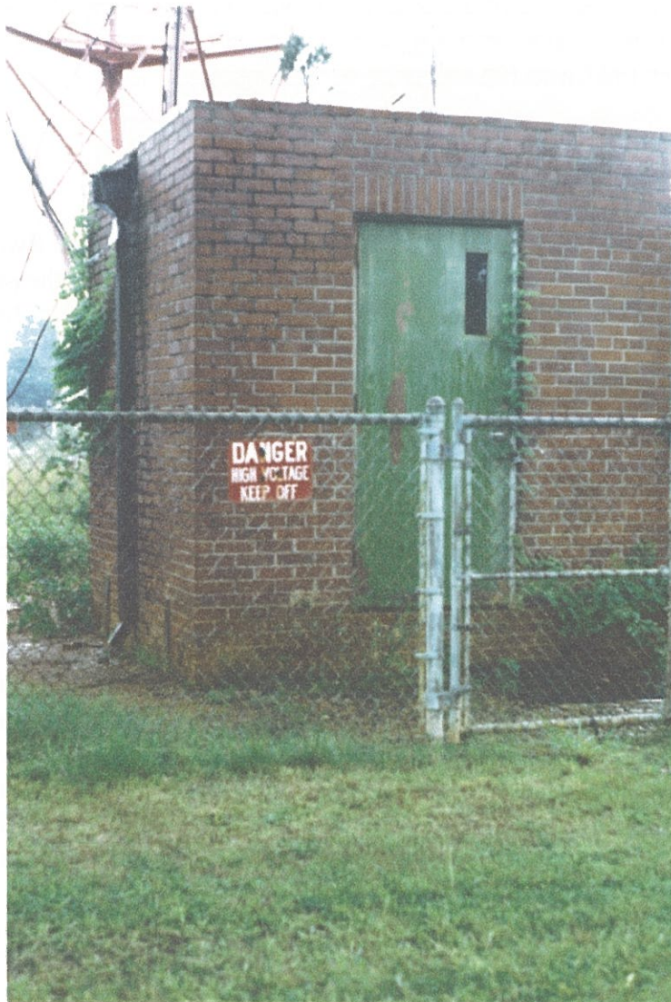
This radio equipment building, better known in radio jargon as the "dog house", located next to the base of the original radio antenna tower of WANK is the only one, as with the tower, of the original five still standing today. This small building was erected in 1937 to house the antenna tuning units for the old AM system, while the transmitters were located inside the main building of each radio station. When the network switched from AM to FM systems in 1945, the new FM transmitters were installed in these smaller buildings. Photo taken 27 June 1995
