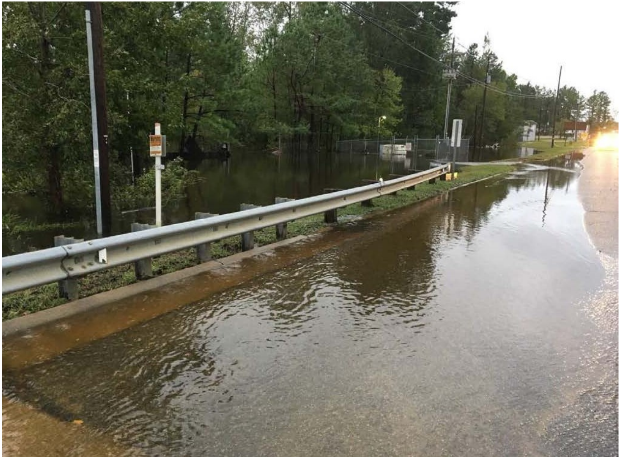
N. Walnut Street pump station site during Hurricane Florence flooding / Note station on left of highway and site completely underwater, days following Hurricane Florence
