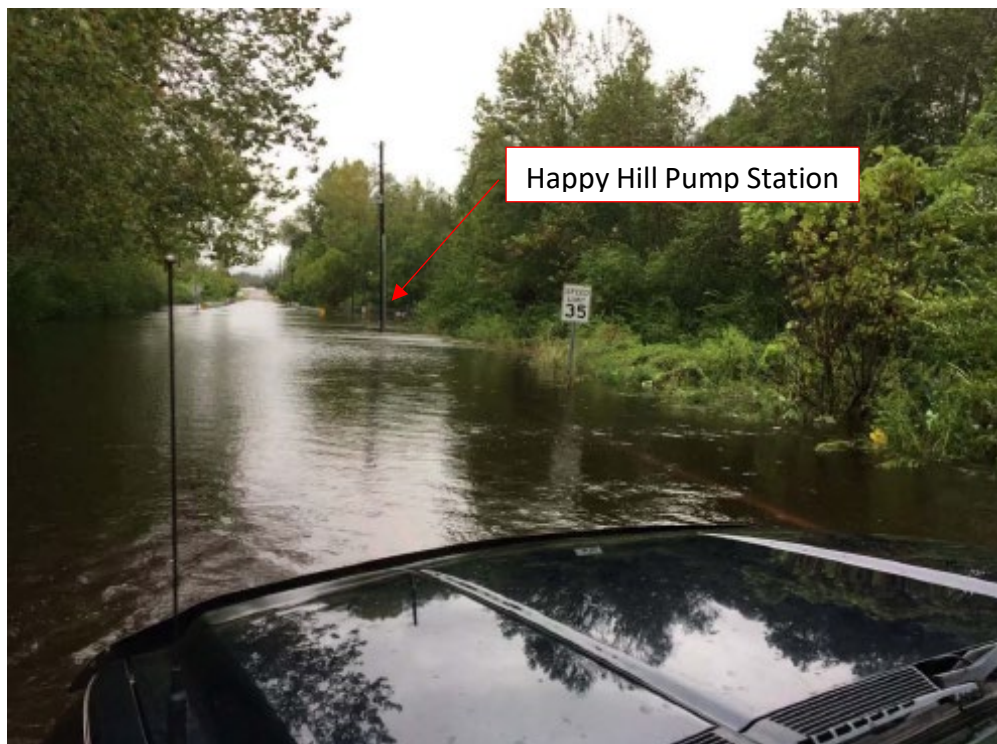
Figure 2.1 Happy Hills Pump Station During Hurricane Florence
