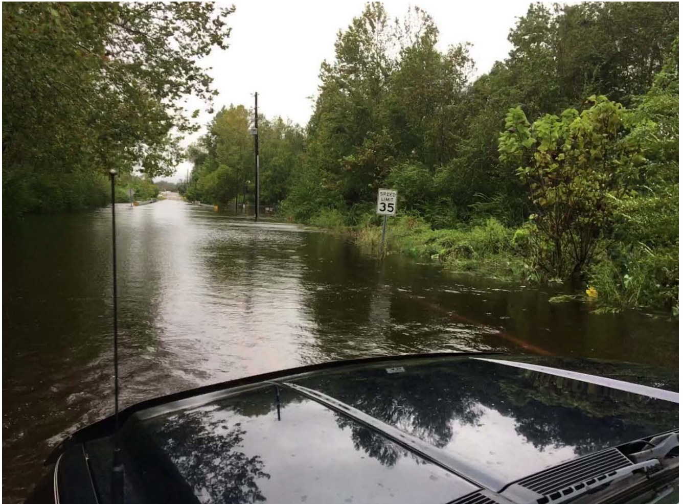
Happy Hill Pump Station – The flooded pump station is seen in the background following Hurricane Florence with no access to the station, located near the utility pole in center of picture
