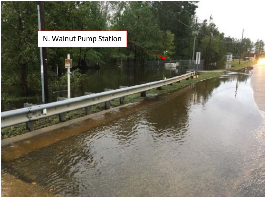
Figure 2.2 North Walnut Pump Station During Hurricane Florence
