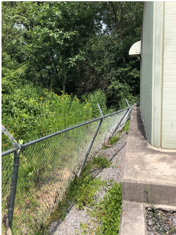
Evidence of Flooding - Damage to Fencing and Floating Debris Deposits
