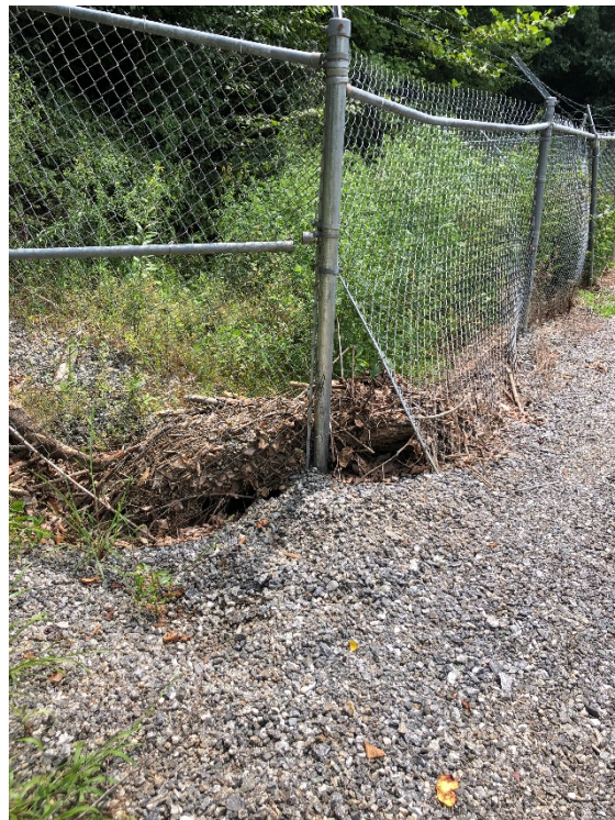
Evidence of Flooding - Damage to Fencing and Floating Debris Deposits
