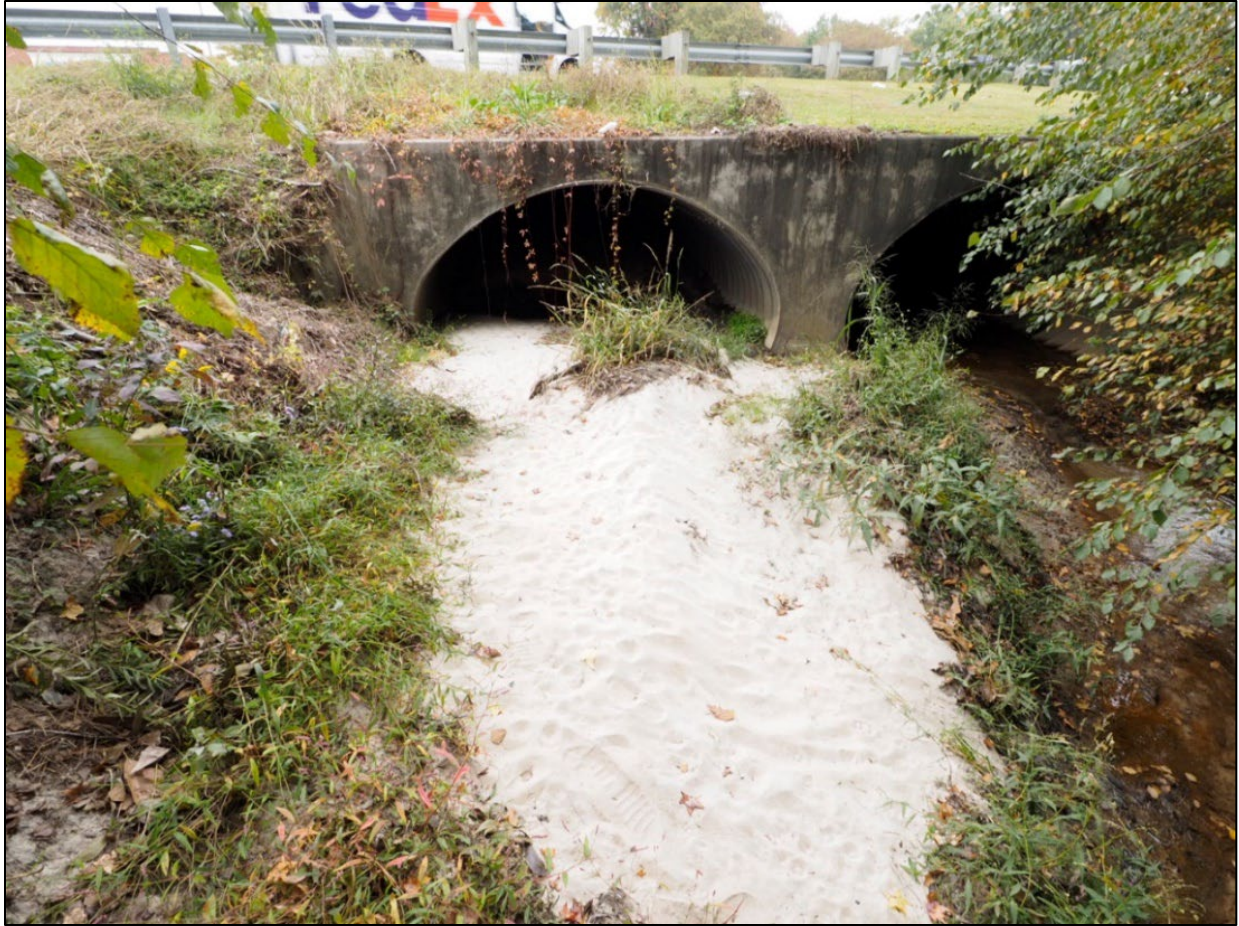
Figure 1. Existing FSUT3 Culvert Pipes at E. Fire Tower Rd. – Downstream Face.
