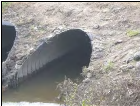
Picture 3-5. Trafalgar Drive – North Culvert – Downstream Face
