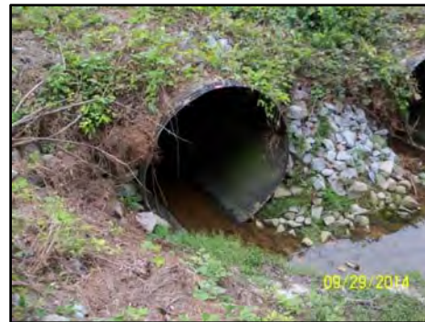
Picture 3-2. Railroad Crossing Culvert – Upstream Face
