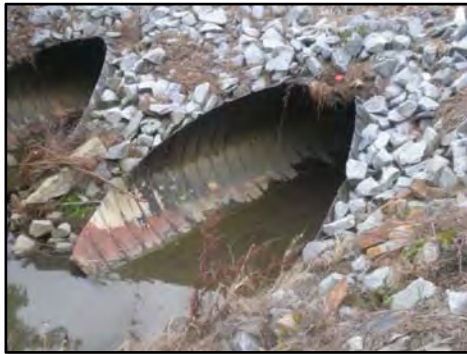
Picture 3-11. Wimbledon Drive Culvert – Upstream Face
