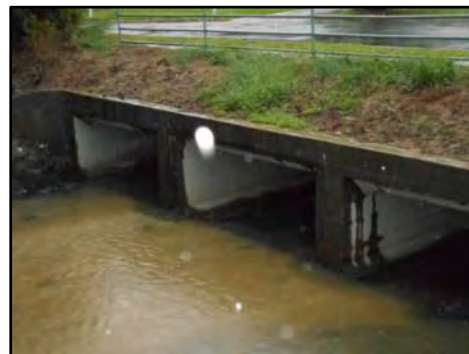
Picture 3-8. Coleman Drive Culvert – Downstream Face
