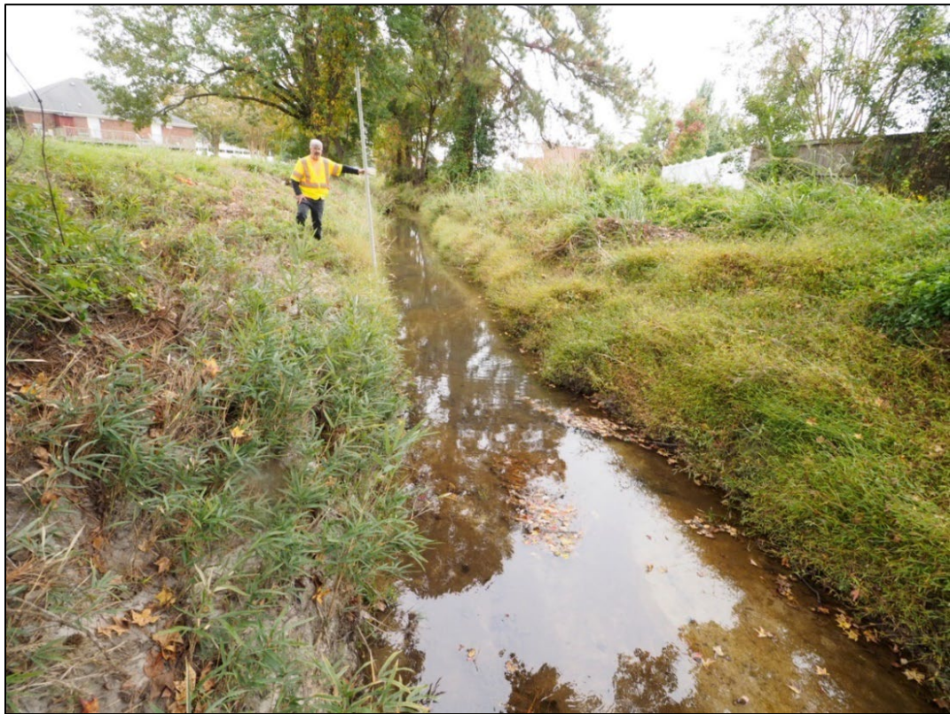
Figure 4. FSUT3 Cross Section #2, Upstream of E. Fire Tower Rd. – 9 feet deep, 8 feet wide.
