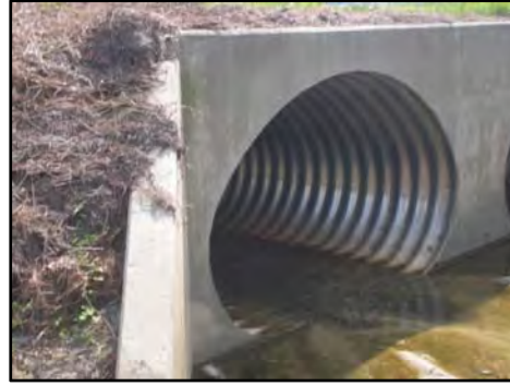
Picture 3-14. East Tower Road –D/S Culvert – Upstream Face
