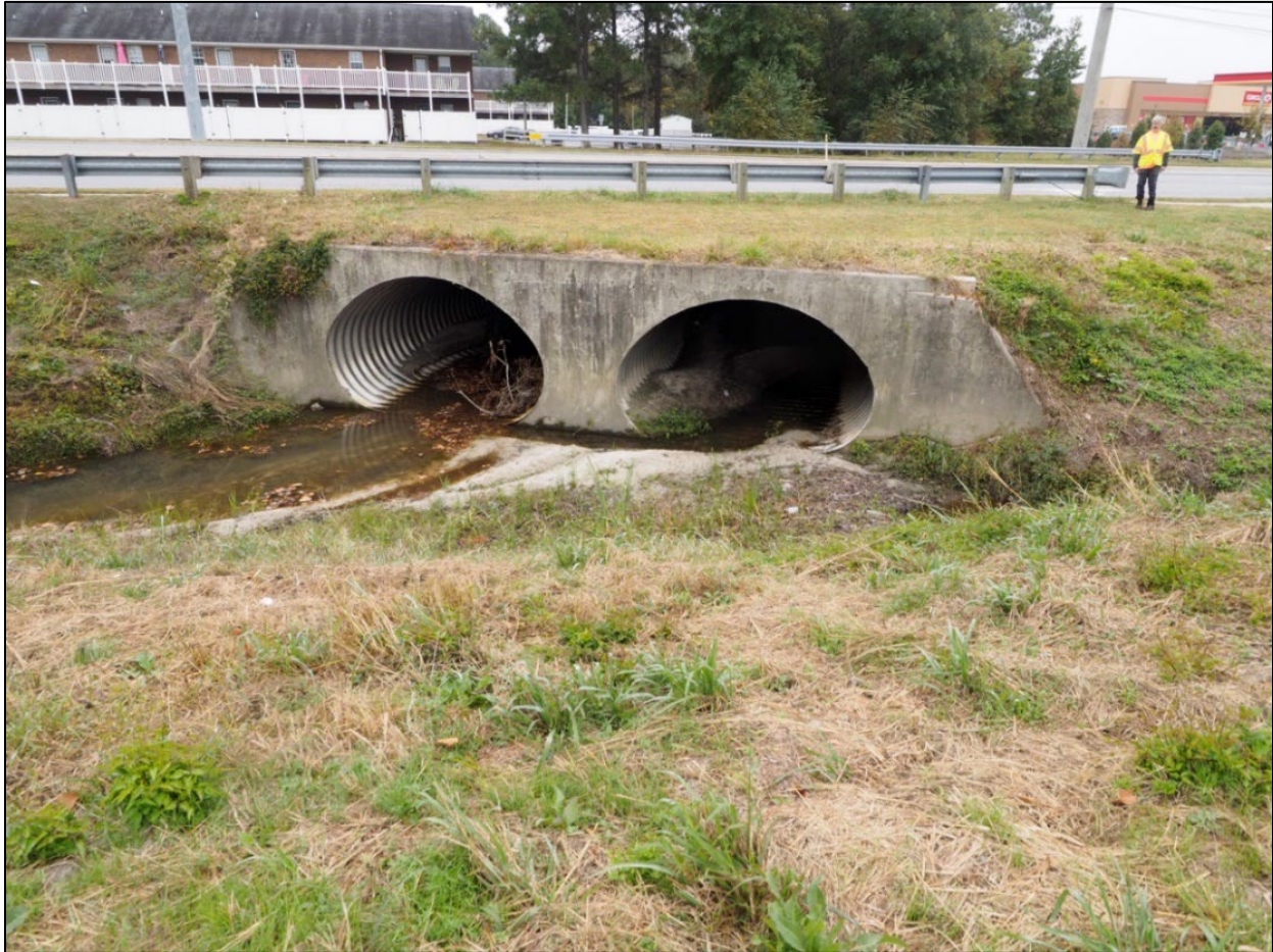
Figure 1. Existing FSUT3 Culvert Pipes at E. Fire Tower Rd. – Upstream Face.
