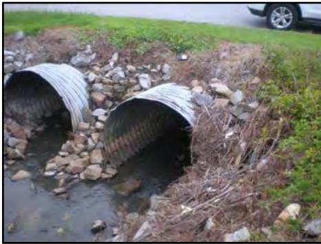
Picture 3-13. Summerhaven Drive Culvert – Upstream Face
