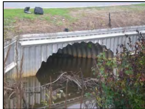
Picture 3-6. Corey Road Culvert – Upstream Face
