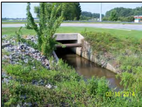
Picture 3-7. West Fire Tower Road Culvert – Downstream Face
