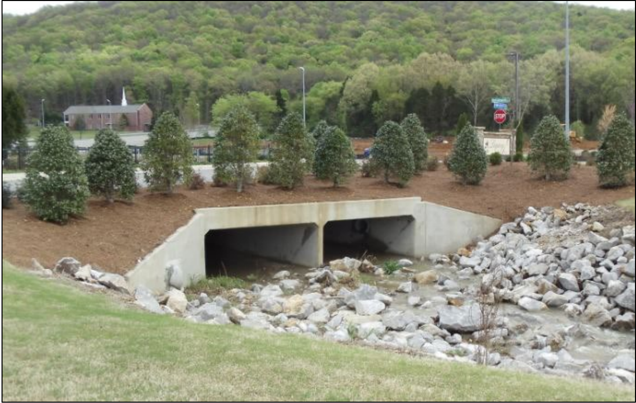
Figure 9. Example Large-Scale Double Culvert Structure
