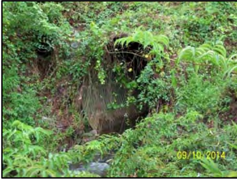
Picture 3-3. Evans Street Culvert – Downstream Face
