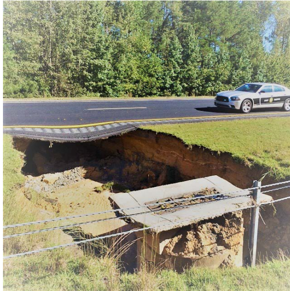
FIGURE 5.13: SINKHOLE IN NORTH CAROLINA
