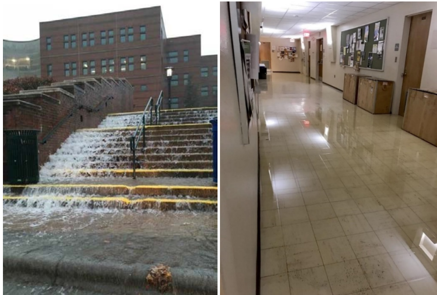
FIGURE A.26: CAMPUS FLOODING (OCTOBER 23, 2017)
